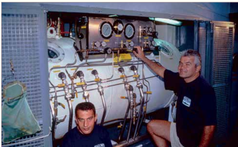
The multi-place, double-lock hyperbaric chamber in MV Saros. Hasan Gül and Dr Akın Savaş Toklu (right) at the recompression chamber on board MV Saros during the two excursions in 1997/98 to identify AE2 (Photo Mark Spencer).
